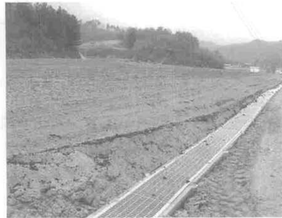
(b) Drainage ditch
